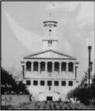
STATE CAPITOL BUILDING
